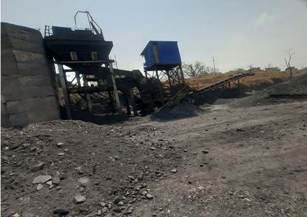
Hopper in the railway siding area
