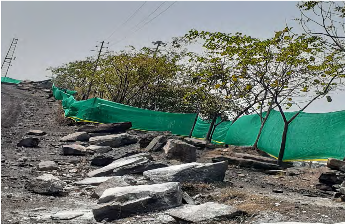
Green belt at the hopper near the railway siding.
