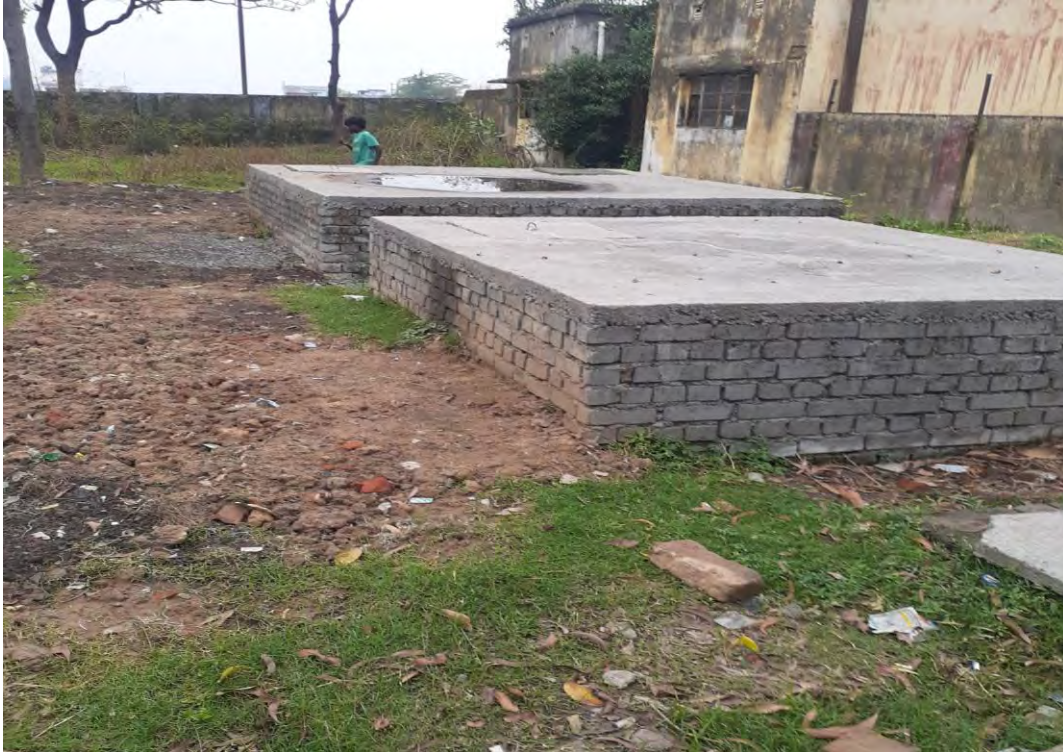
Rainwater harvesting structure
