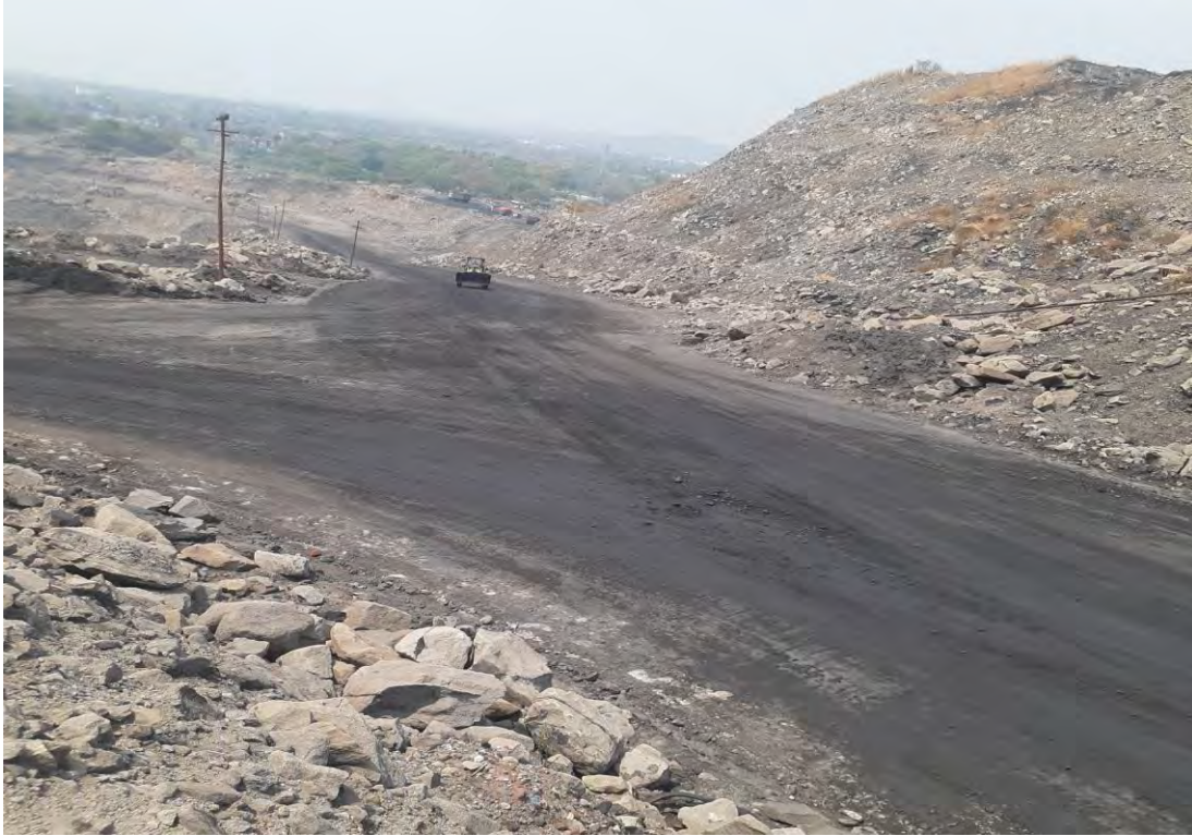
Internal road and active OB dump in Ghondudih Khas Kusunda opencast mine
