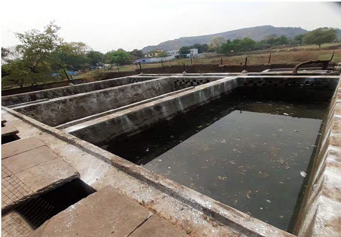
Mine Water treatment plant
