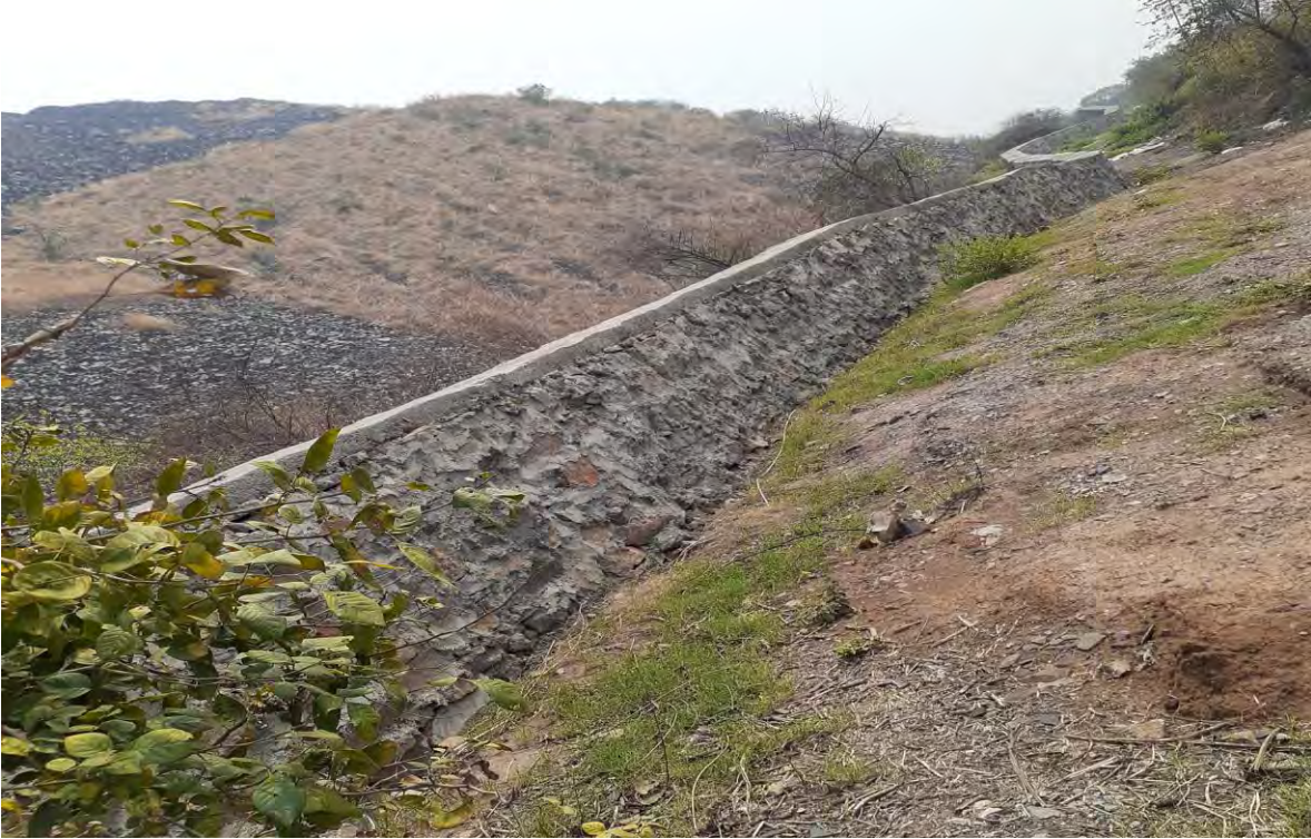
Toe wall and catch drain around the stabilized OB dump in Godhur opencast coal mine area
